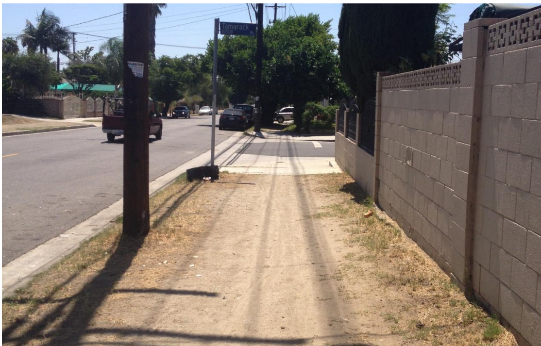
SIDEWALK ABRUPTLY ENDS MULTIPLE TIMES ALONG PIERCE STREET
