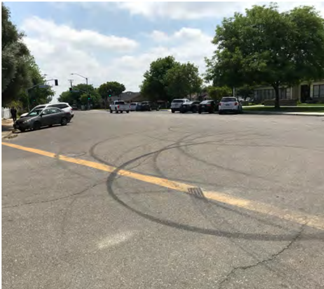
Left: Tire markings at Spruce Street and South Avenue.
