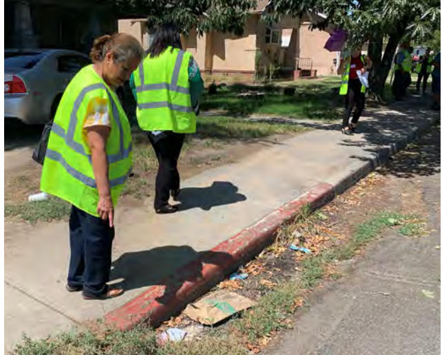
A participant inspects a gutter clogged with debris and overgrown weeds on South Orange Street.
