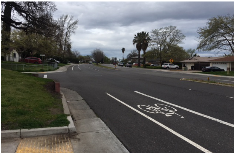
Views of the intersection of Hillsdale Boulevard and Diablo Drive where a sidewalk ends in a bike lane and forces pedestrians to walk into the street to cross at Diablo Drive. Photo: California Walks and UCB SafeTREC
