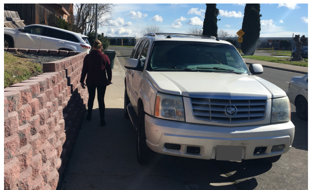
A driver uses the rolled curb to drive up onto the sidewalk, reduces the sidewalk width, impacts walkability, and blocks sidewalk access for people using assisted mobility devices, such as wheelchairs. Photo: California Walks
