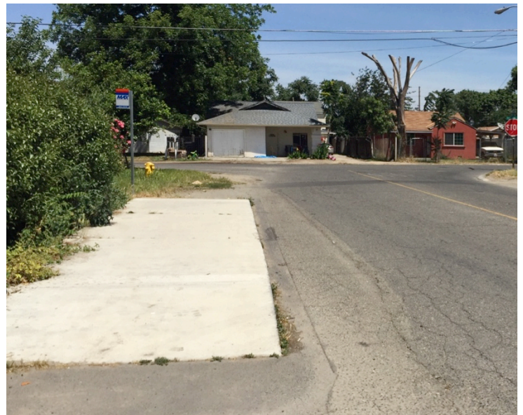
EXAMPLE OF EXISTING BUS STOP THAT HAS NO SHELTER AND DOES NOT CONNECT TO SIDEWALKS
