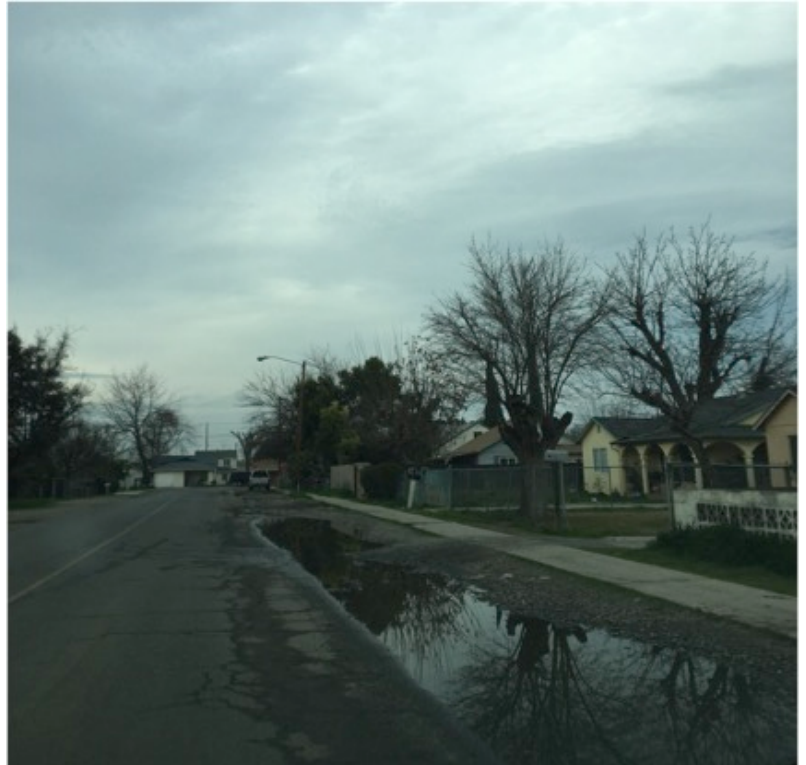
POOR DRAINAGE SYSTEMS LEADING TO LARGE PUDDLES
