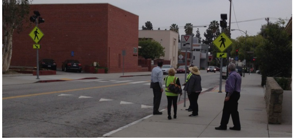
NEW HIGH-VISIBILITY MID-BLOCK CROSSWALK WITH ACCOMPANYING SIGNAGE, BEACONS, AND ADVANCE YIELD LINES.
