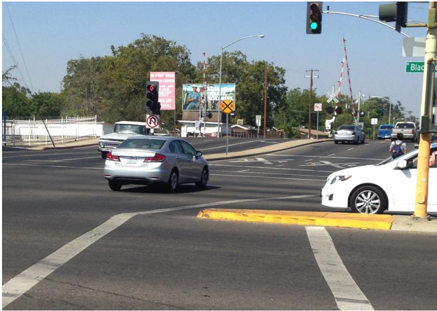
TRAFFIC MEDIAN OBSTRUCTS CROSSWALK ON BLACKSTONE AVENUE
