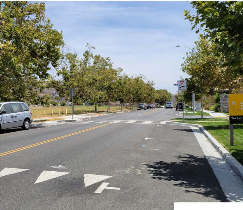
LEFT: Bulb-outs, planting strips, and continental crosswalk markings on River Street.
