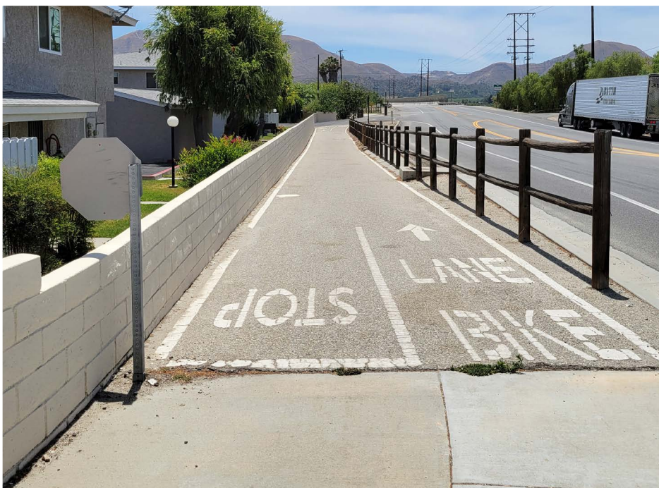
LEFT: The bike path on SR-23 that ends abruptly.
