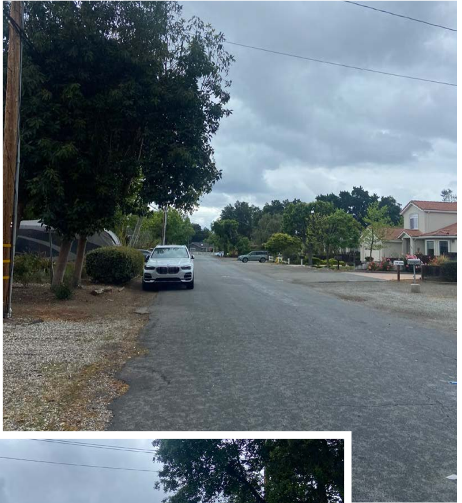
BELOW: Missing sidewalks in both directions on Regina Way.
