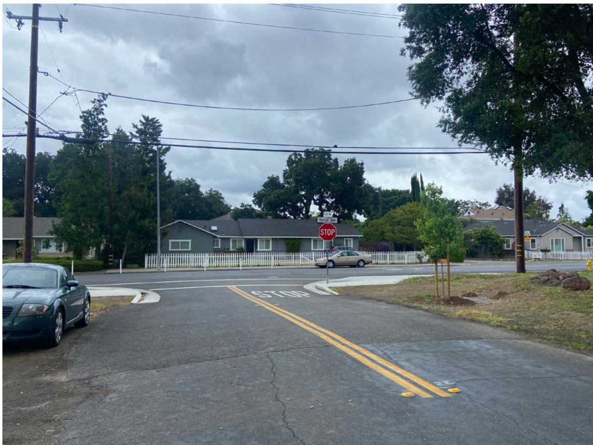
ABOVE: The T-intersection of Regina Way/Harriet Avenue features a standard crosswalk which leads to unpaved shoulders.
