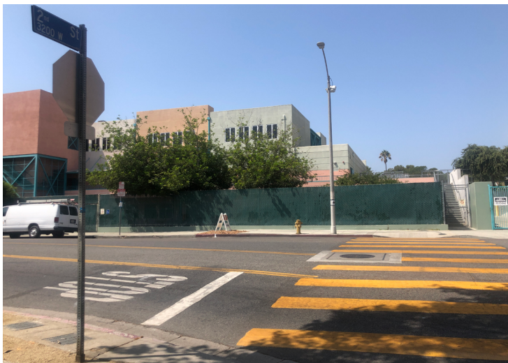
TOP RIGHT: Commonwealth Avenue/4th Street intersection with median stop sign. BOTTOM LEFT: The primary entrance at Commonwealth Elementary.
