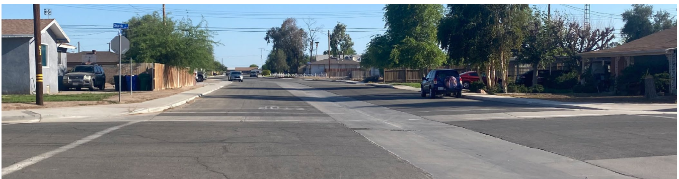
TOP LEFT: Despite the 40 miles per hour speed limit sign posted on Sorensen Avenue (SR-111), at the northern entrance to Calipatria city limits, participants report that drivers often speed when driving through town. TOP RIGHT: The western side of Sorensen (SR-111) south of Bonita Street is a dirt road with trees that impede pedestrian access without providing shade. BOTTOM: Standard transverse crosswalk markings are faded at the Church Street/Park Avenue intersection adjacent to the many churches in this area.
