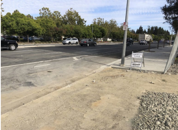
Sidewalk on west side of Oakland Road abruptly ends south of the railroad tracks.
