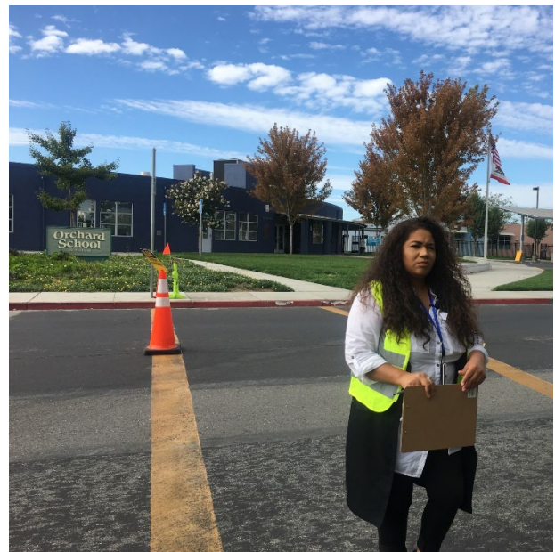
The crosswalk in front of Orchard School lacks enhancements, including a curb ramp on the school side and high-visibility markings.
