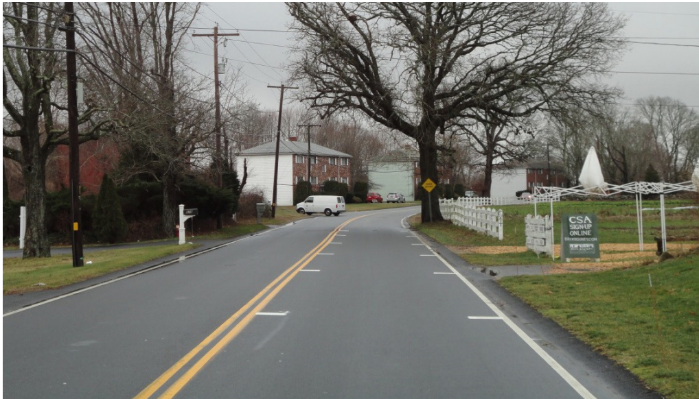
Optical speed bars on a rural road. Source: Federal Highway Administration; Photo Credit: KLS Engineering, LLC
