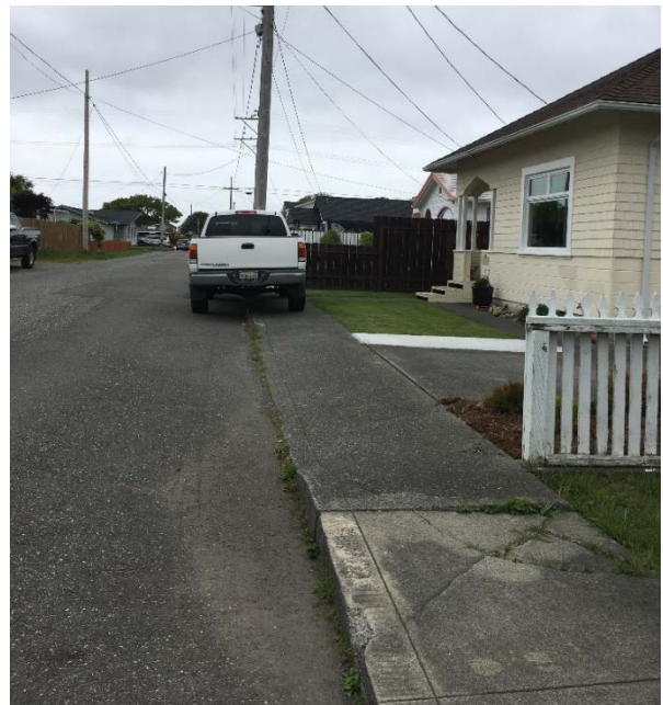
A vehicle parked on the sidewalk along County Lane blocks access for pedestrians. In the right foreground the sidewalk is cracked. Photo Credit: California Walks
