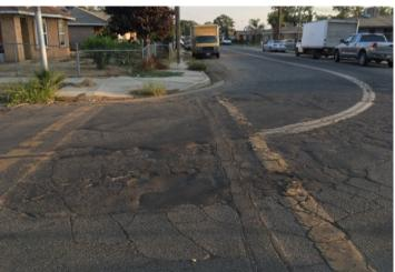
Deteriorating pavement quality and faded markings at S. Santa Clara Avenue & E. Chester Avenue
