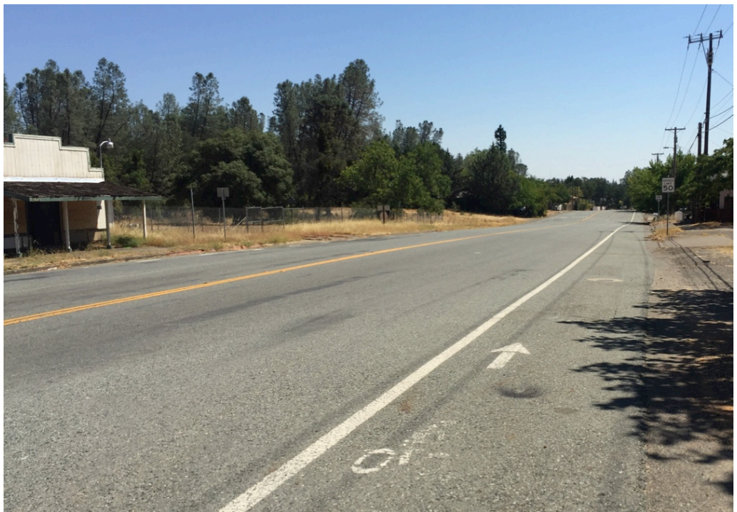
LAKE BOULEVARD NEAR PUBLIC SCHOOL WITH POSTED 50 MPH SPEED LIMIT, NO SIDEWALKS, AND FADED SHOULDER BICYCLE LANE.
