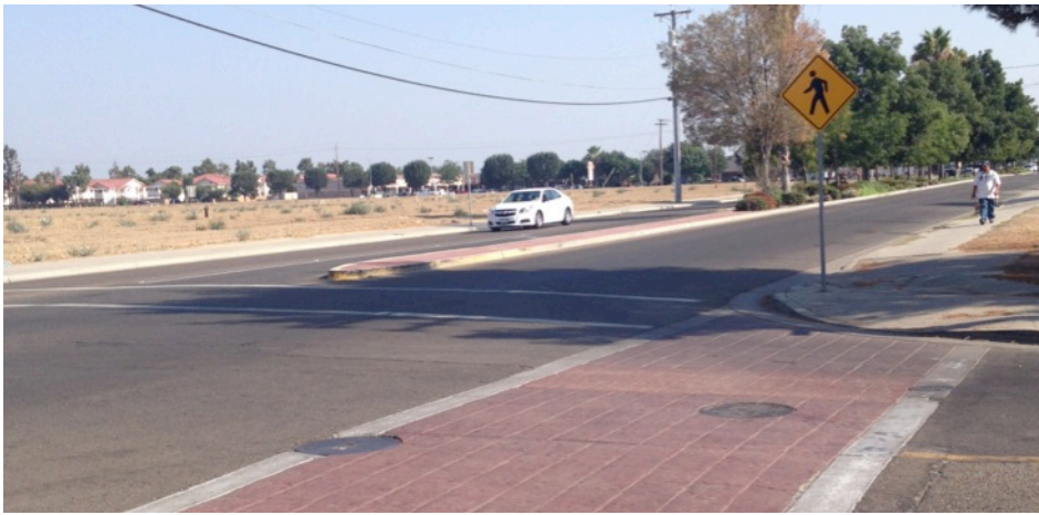
MENDOCINO AVENUE LOOKING SOUTHBOUND AT RECENTLY INSTALLED CROSSWALK AND SIGNAGE AT TUOLUMNE STREET/MULBERRY LANE
