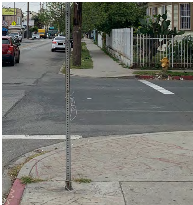
Left: Lack of curb ramps on alleyway. Right: Lack of truncated dome and accessibility features for visually impaired pedestrians at East 25th Street and Hooper Avenue.
