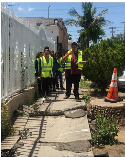
Top Left: Broken sidewalks lifted by tree roots along Whittier Boulevard. Photo: California Walks Bottom Left: Empty tree well along East 6th Street, in front of Hollenbeck Middle School creates uneven walking surface and tripping hazard. Photo: California Walks
