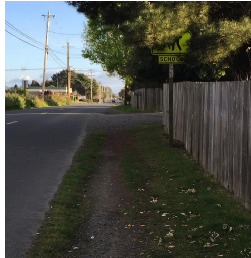
OBSCURED SCHOOL ZONE SIGNAGE ADJACENT TO WELL-WORN PEDESTRIAN PATH
