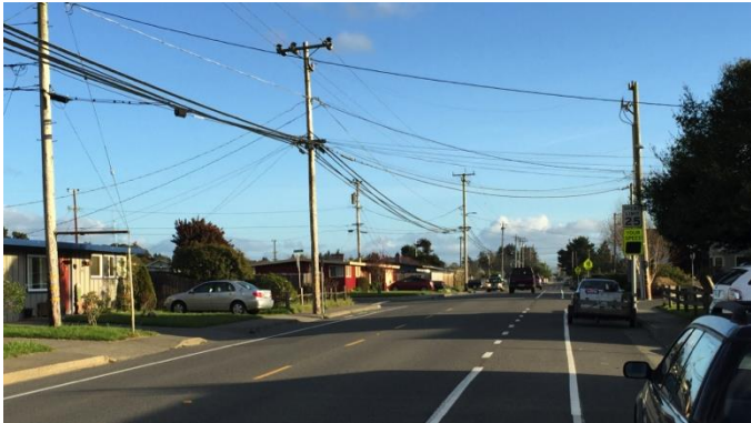
RECENT IMPROVEMENTS TO MCKINLEYVILLE AVENUE SOUTH OF MURRAY ROAD INCLUDE BIKE LANES, SPEED FEEDBACK SIGNS, HIGH-VISIBILITY CROSSWALK MARKINGS AND CONTINUOUS, LEVEL SIDEWALKS.
