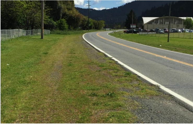
CLEARLY WORN PEDESTRIAN PATHS ALONG BOTH SIDES OF SR-96 NEAR THE ELEMENTARY AND HIGH SCHOOLS
