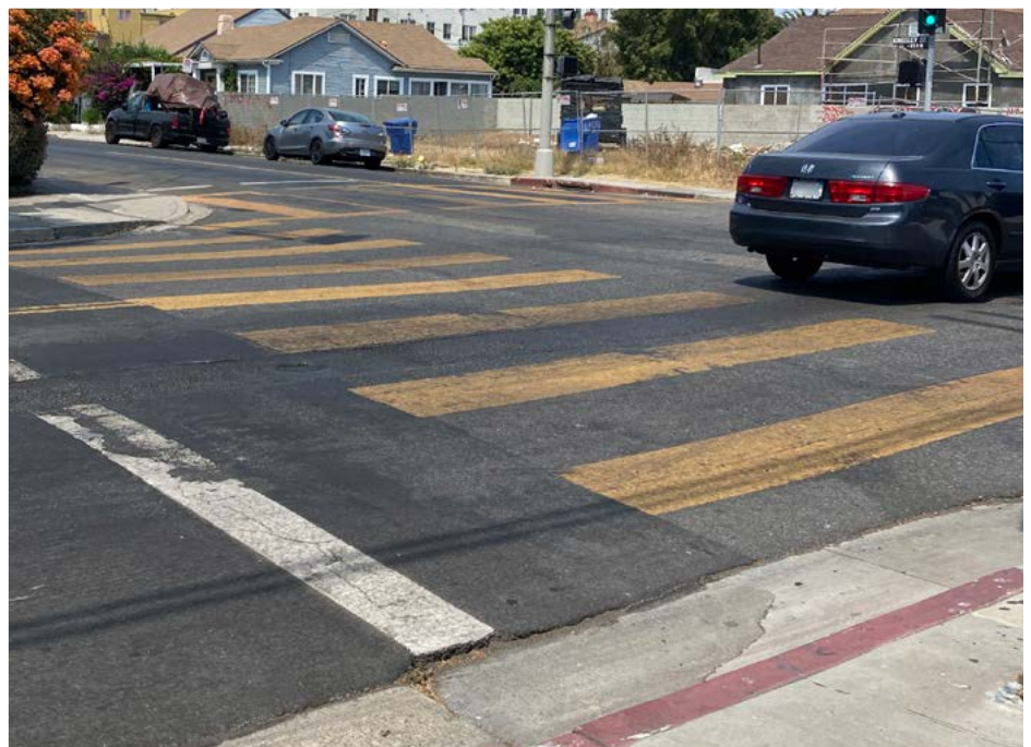
RIGHT: An example of daylighting at Oakwood Avenue/ N Kingsley Drive.
