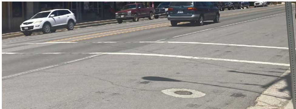
Faded crosswalk markings in front of Five Marys Restaurant and Mechanics Bank
