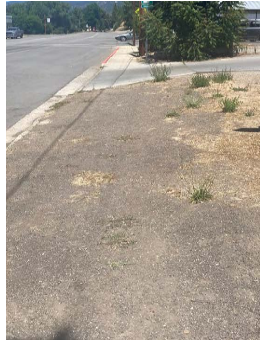
Uneven gravel by the U.S. Post Office
