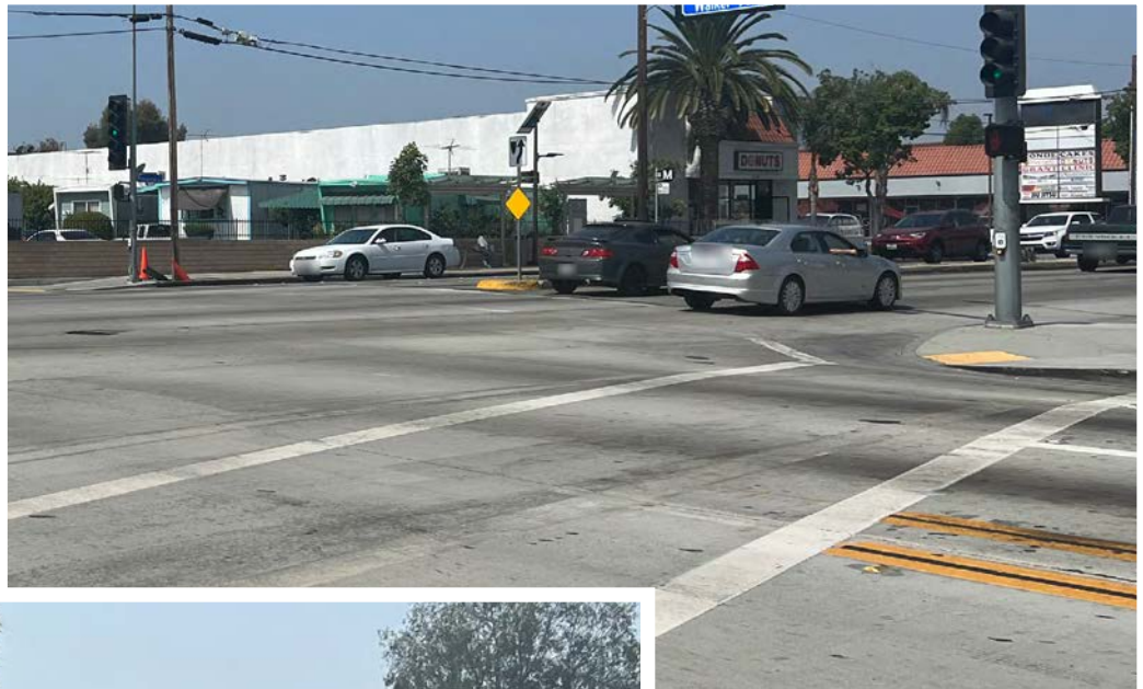
Top: The East Florence/ Walker Avenue intersection, next to the new Bell park, has standard marked crosswalks and is four lanes wide with short crossing times.
