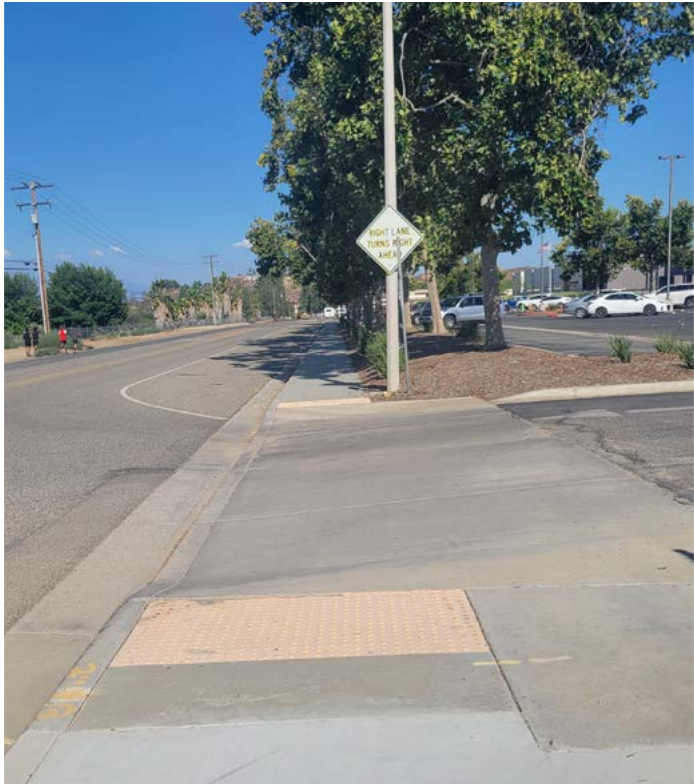
ABOVE: Truncated domes in front of MVMS alert pedestrians of a driveway where vehicles may be present.
