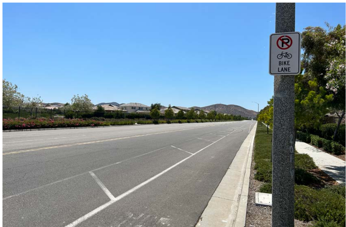
BELOW: View from Craig Avenue looking south towards Evans Road, including a sidewalk and bike lane
