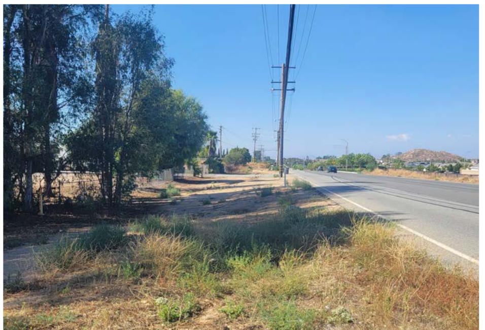
RIGHT: Wide dirt shoulders where people walk on Murrieta Road with overgrown weeds and debris.
