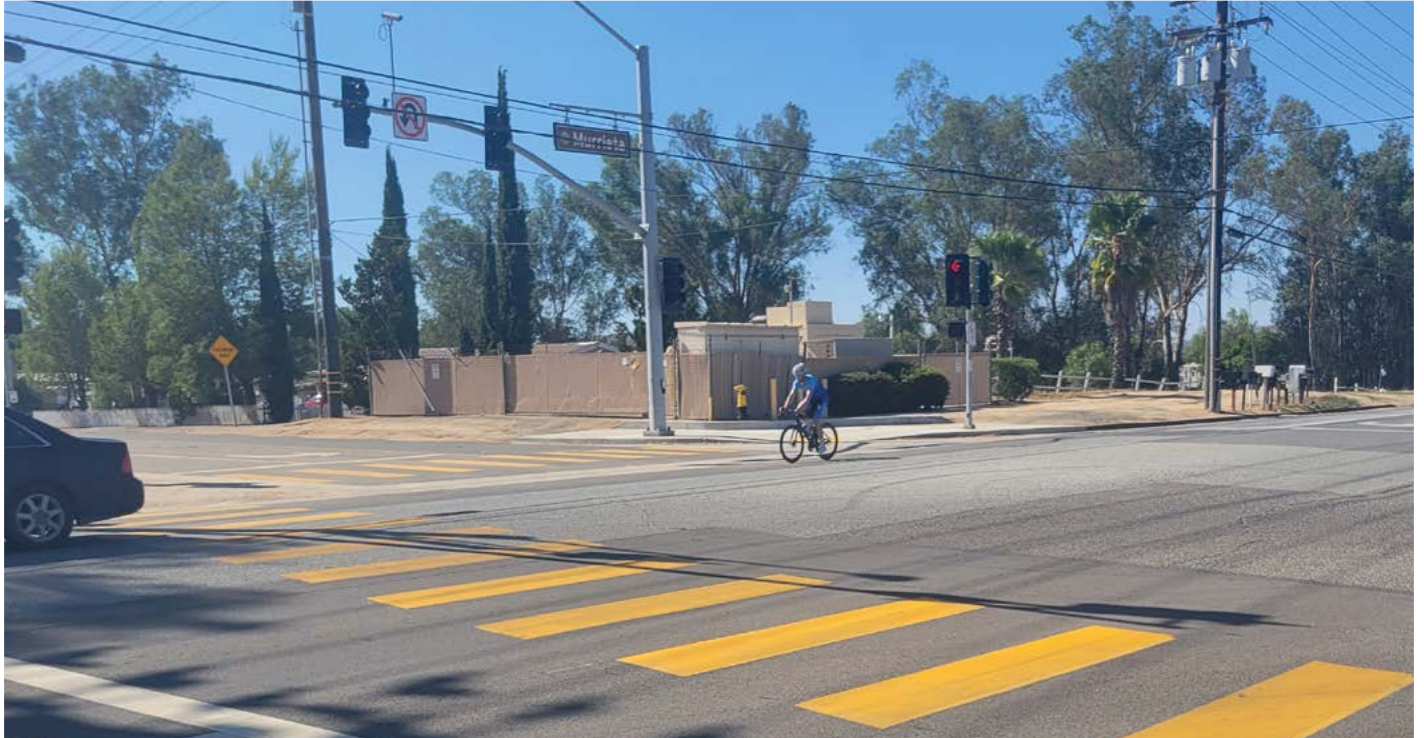
ABOVE: A bicyclist crossing the Murrieta Road/Garbani Road intersection where crosswalks are painted with continental markings.
