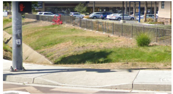
The sidewalk on the Southwest corner of 17th Street/Newport Boulevard, in front of Chase, is narrow and forces wheelchair users to wait on the street to cross the intersection.
