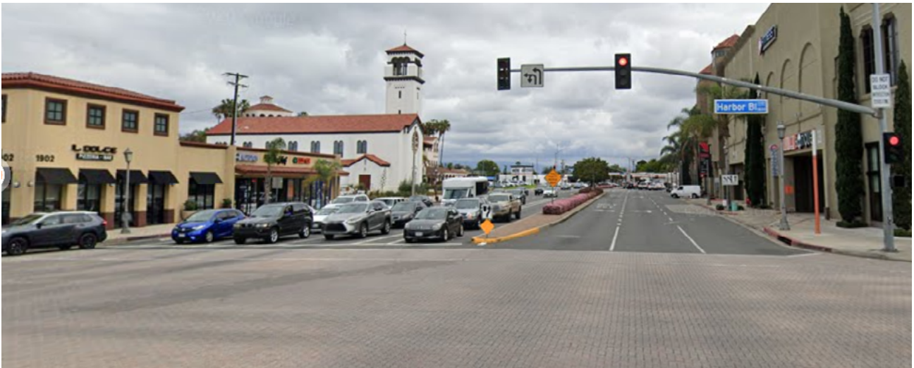
Crosswalk along Harbor Boulevard at the 19th Street/ Harbor Boulevard intersection is 8 lanes wide and pedestrians do not feel there is enough time to cross in a safe and calm manner.
