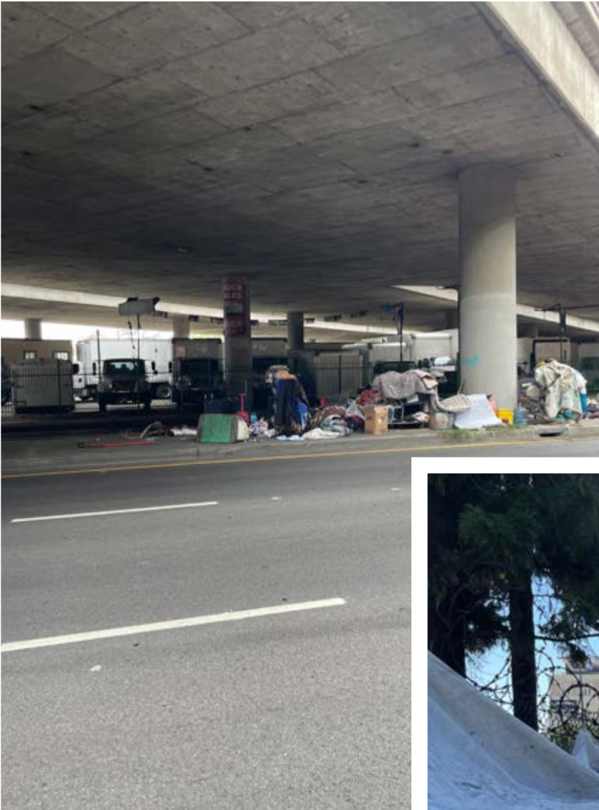
ABOVE: The section under the freeway bridge on West Washington Boulevard tends to be dark, making it dangerous at night and early morning.
