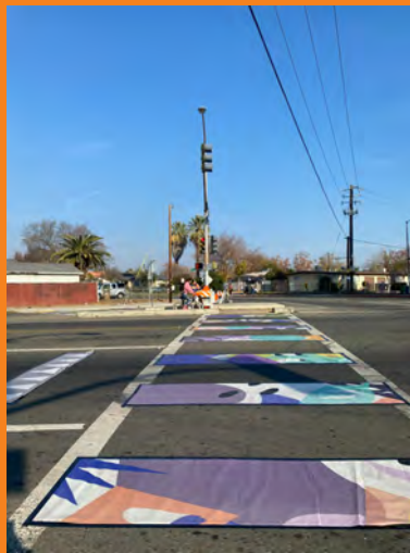
IMAGE: INSTALLED TEMPORARY CREATIVE CROSSWALK
