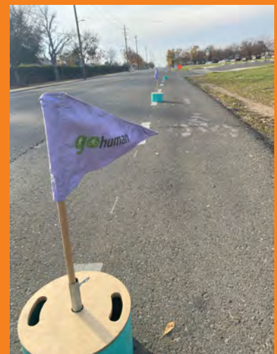
IMAGE: SOUTHERN CALIFORNIA ASSOCIATION OF GOVERNMENTS GO HUMAN KIT OF PARTS PROTECTED BIKE LANE MATERIALS
