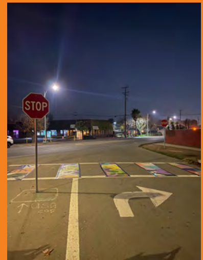
IMAGE: CREATIVE CROSSWALK INSTALLED OVER AN EXISTING MARKED CROSSWALK IN A RIGHT-TURN SLIP (SEPARATED) LANE
