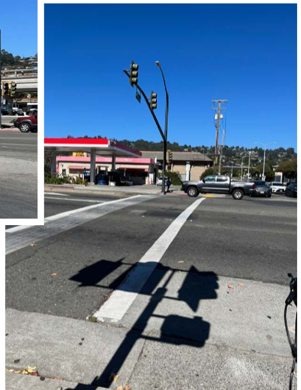
TOP LEFT: Unmarked crosswalk on the north end of the San Pablo Avenue/Hill Street/Eastshore Boulevard/Peerless Avenue five-way intersection. BOTTOM RIGHT: Crossing at the north end of the San Pablo Avenue/Moeser Lane intersection.
