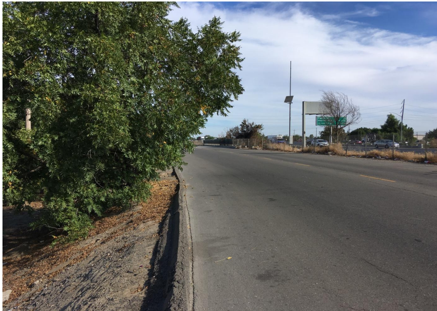
Traveling northbound on Manthey Road, the foot path on the west side becomes un navigable, forcing residents to walk in the street where they are obscured from oncoming traffic by overgrown vegetation.
