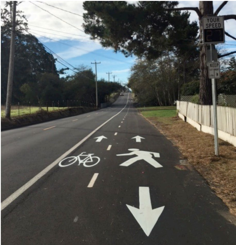
Example of a pedestrian lane treatment in McKinleyville, CA. Population: 15,177. Photo Credit: Redwood Community Action Agency.
