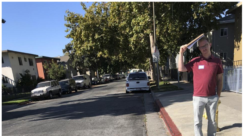
At Appian Lane and McLaughlin Avenue approaching McKinley Elementary, there is only one small speed limit sign which is partially obscured by a smaller parking sign. There are no road markings and no school zone signage.
