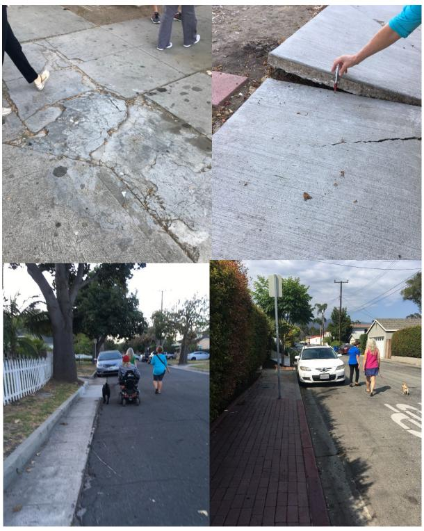
Missing, narrow, upheaved, and cracked sidewalks in the Westside.
