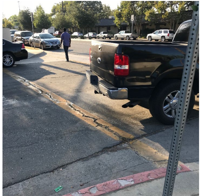
Parents parking in the no parking zone along Woodbury road at Spaulding place block visibility of drivers turning right and left onto Woodbury.
