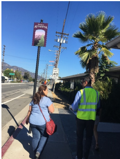
Landmark, speed limit, and construction zone signage limit visibility of school zone signage at Woodbury Road and Canada Avenue.
