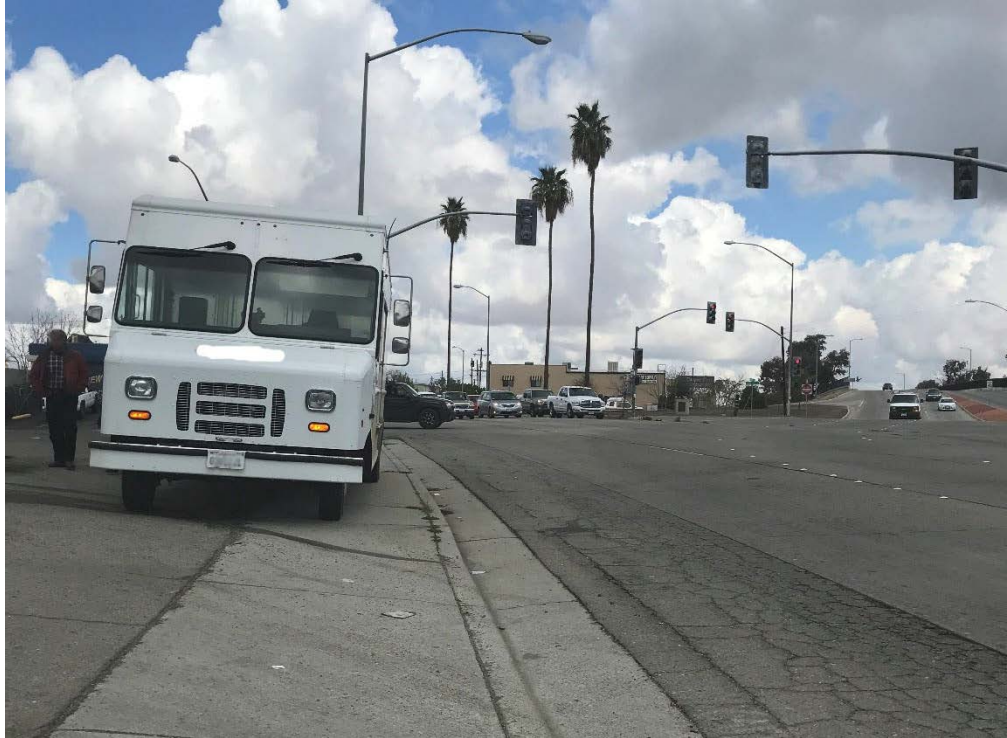
A large truck parked on the sidewalk blocks the pedestrian's right-of-way on a sidewalk along on SR 204.
