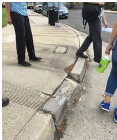
Example of multiple curb ramps that are flush with the street and that lack truncated domes for blind or visually-impaired pedestrians (left) and example of an intersection with a cracked curb and missing curb ramps (right).
