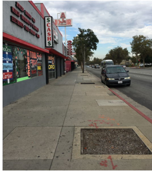
Empty tree wells along Holt Avenue provide no shade to pedestrians and can create challenges to pedestrians with disabilities.
