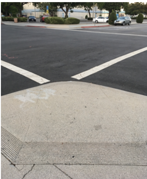
Example of multiple curb ramps that are flush with the street and that lack truncated domes for blind or visually-impaired pedestrians (left) and example of an intersection with a cracked curb and missing curb ramps (right).
