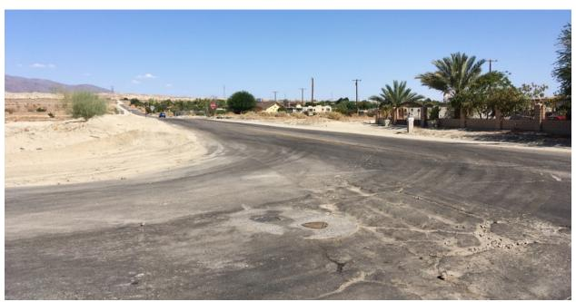
Wide streets with minimal pavement markings. Wide turn radii of streets can encourage drivers to make turns at high speeds.
