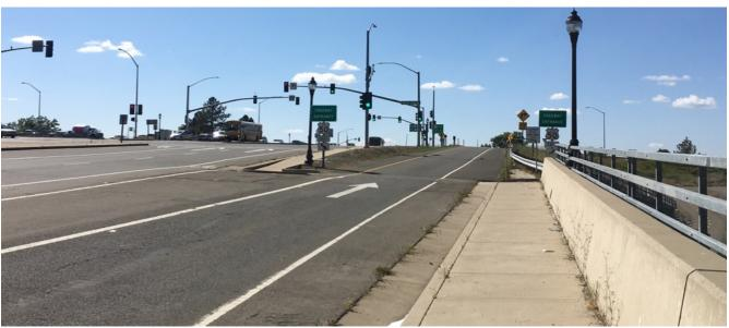
Lack of crosswalk markings or pedestrian warning signage at US 50 on- and off-ramps.
