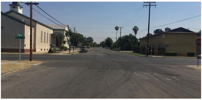
Faded stop sign and stop bar markings.
