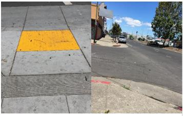
Left: Newer ADA-compliant yellow truncated dome ramp. Right: Older, concrete non-compliant ramp.
